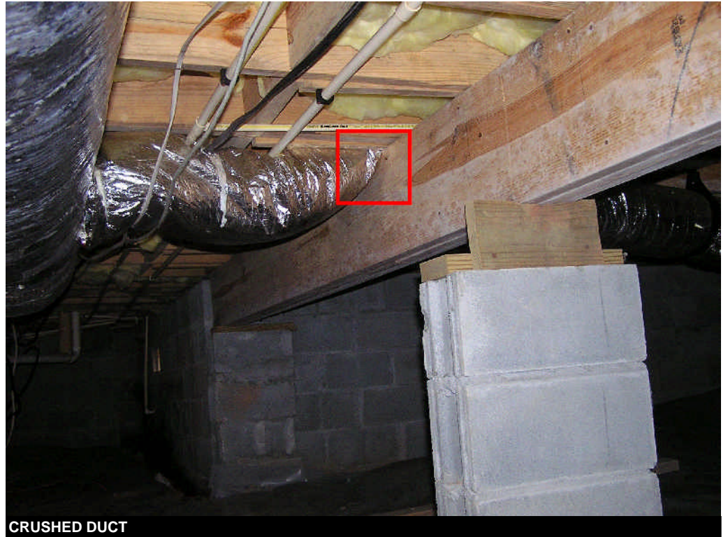
CRUSHED DUCT
